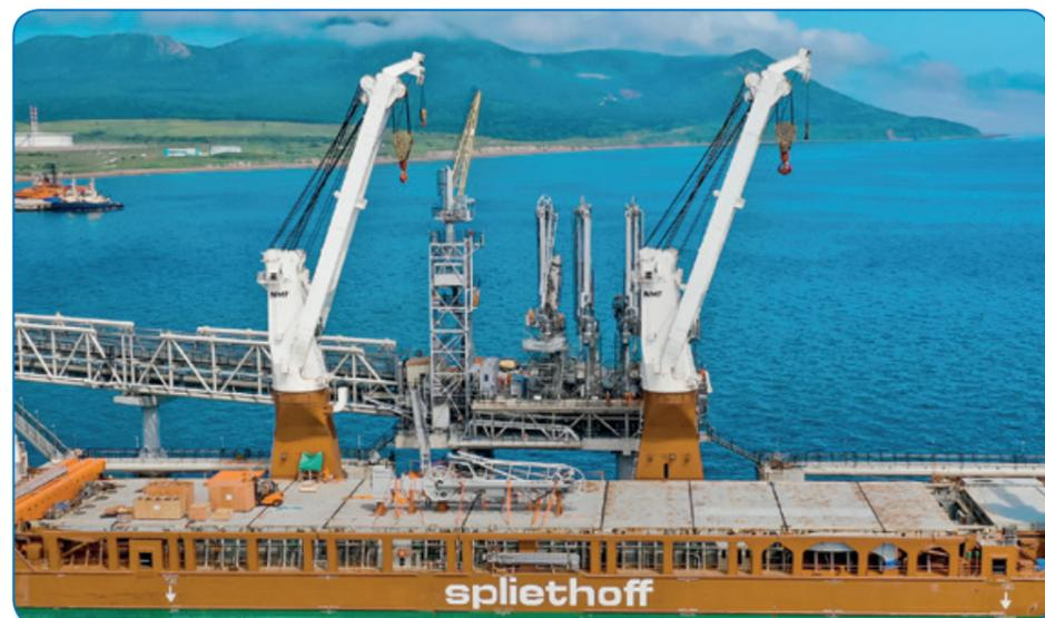
Two of the four loading arms were replaced at the LNG jetty of Prigorodnoye production complex
