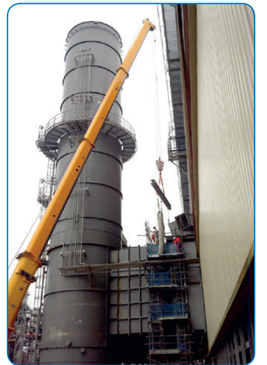
Installation of gas turbine exhaust duct expansion joint
