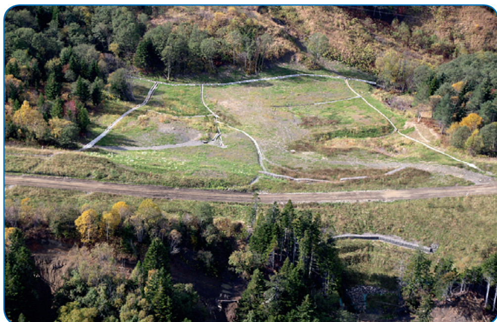
The surface and deep drainage systems on the landslide area
