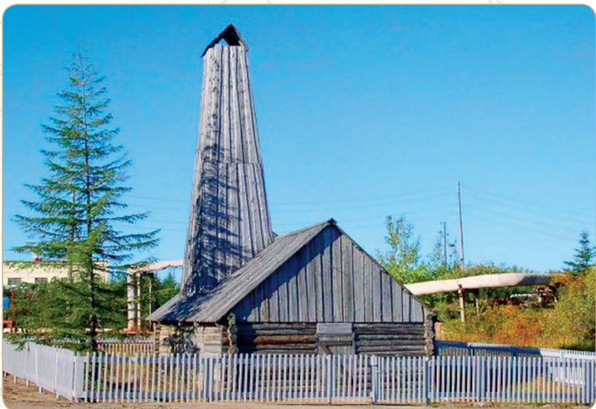
The first industrial oil was produced on Sakhalin on 12 May 1910 under the leadership of Mining Engineer Mindov. For this purpose, a wooden rig was built in the Okha field, which has survived to this day and is now a historical monument. The Zotov rig, used to drill the first industrial well in the region, was operated until the 1950s. Photo courtesy of www.ruspekh.ru
