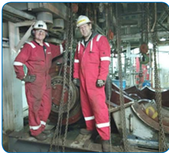
Removal of the bull gear and crankshaft from the existing IDECO 1600 triplex mud pumps that will be replaced with the quadruplex whitestar mud pumps
