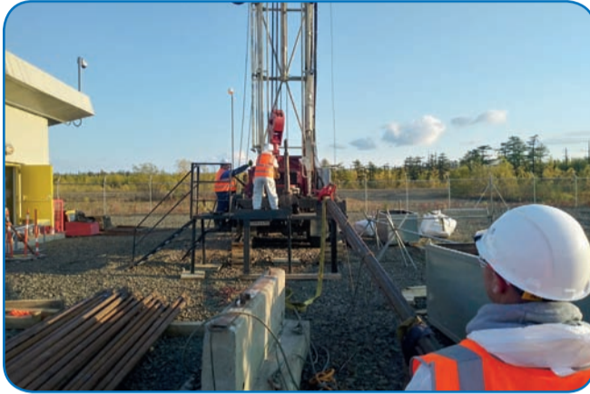
Drilling works at the OPF water intake
