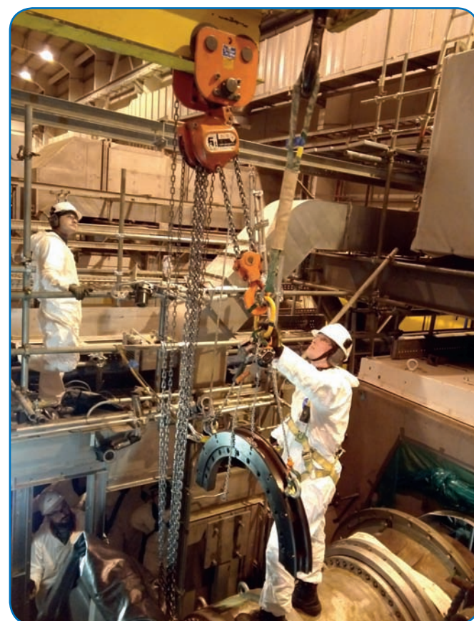
Disassembly of the turbine: the support ring of the first nozzle apparatus is removed
