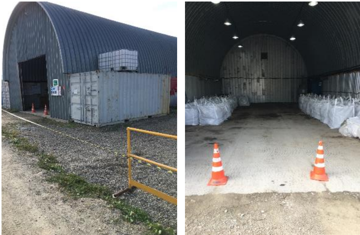
Figure 4.1 - General views of the exterior and interior of the non-hazardous waste storage shed
