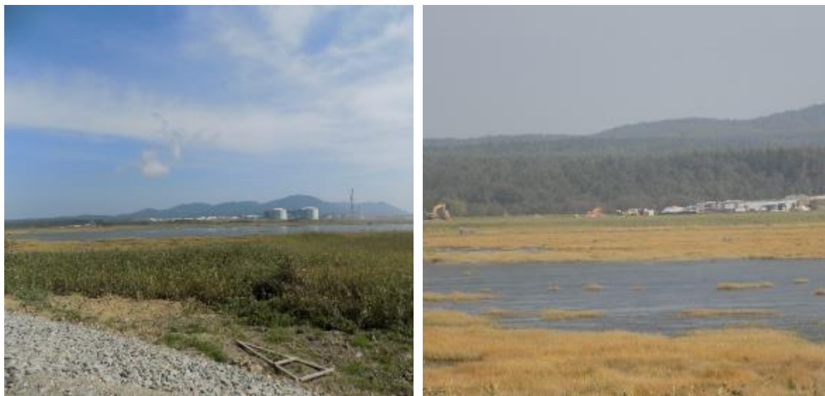
Figure 3.7 – Mereya Wetland, showing proximity to LNG and restarted bridge works
