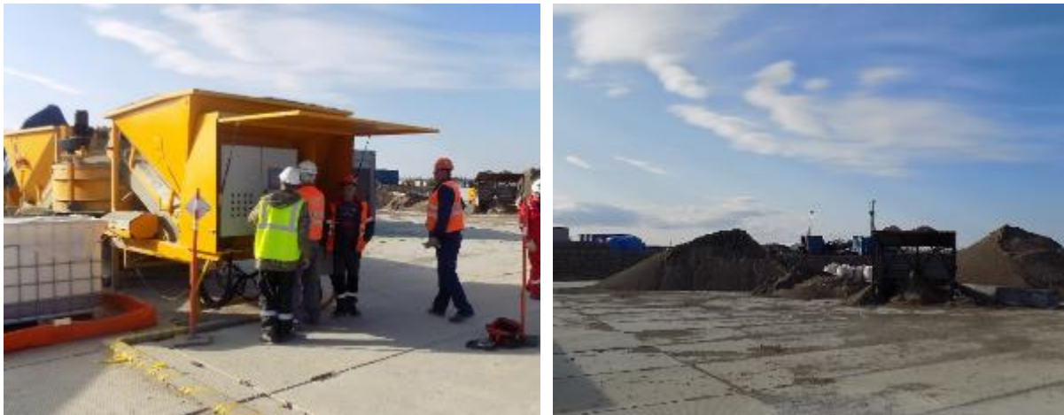
Figure 2.13 – Concrete batching plant and associated storage area on Construction site
