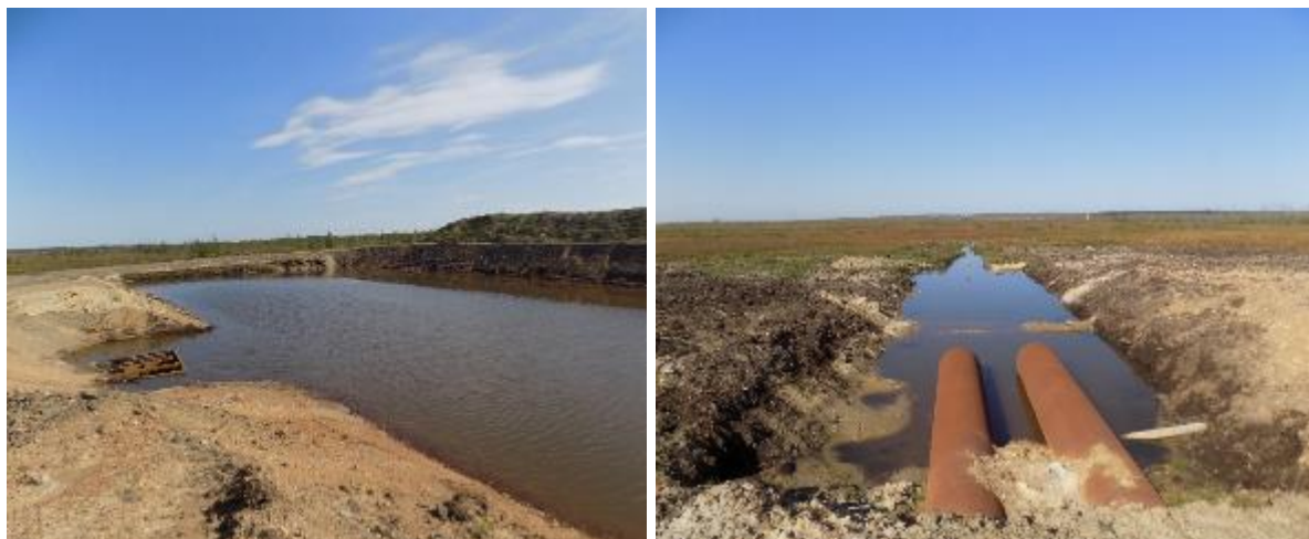
Figure 2.7 – Peat Storage Area Settlement pond and Discharge point
