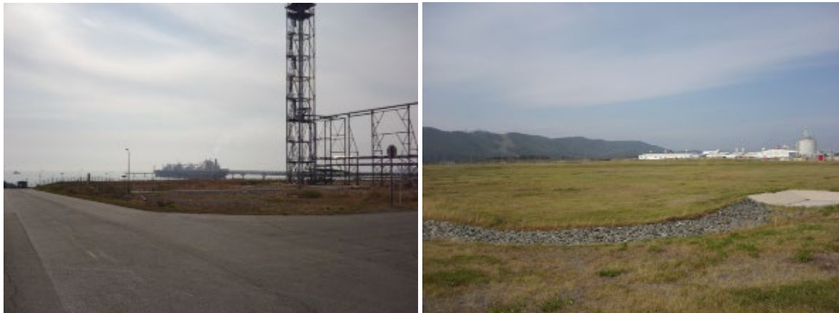
Figure 3.2 - View of the areas earmarked for new LNG loading Jetty (between the MOF and existing LNG loading jetty) and for the new bulk LNG storage tank.
