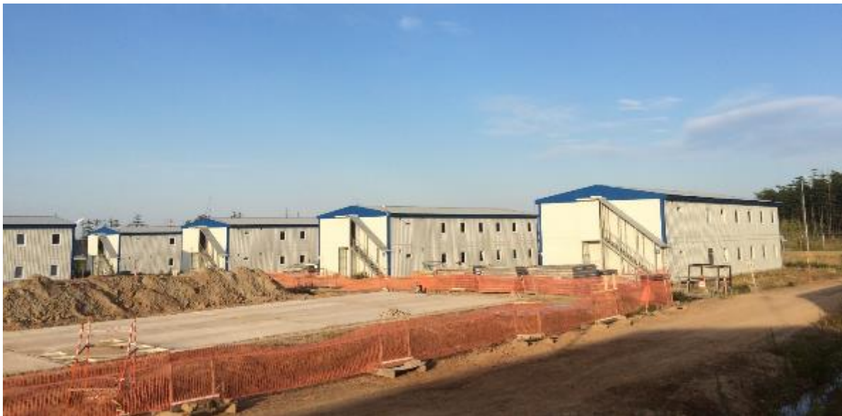
Figure 2.2 Fly camp refurbishment and main camp construction area
