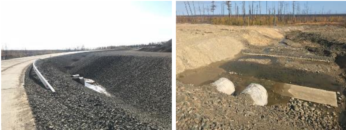
Figure 2.12 – Improved on site water management (photos courtesy of Sakhalin Energy)
