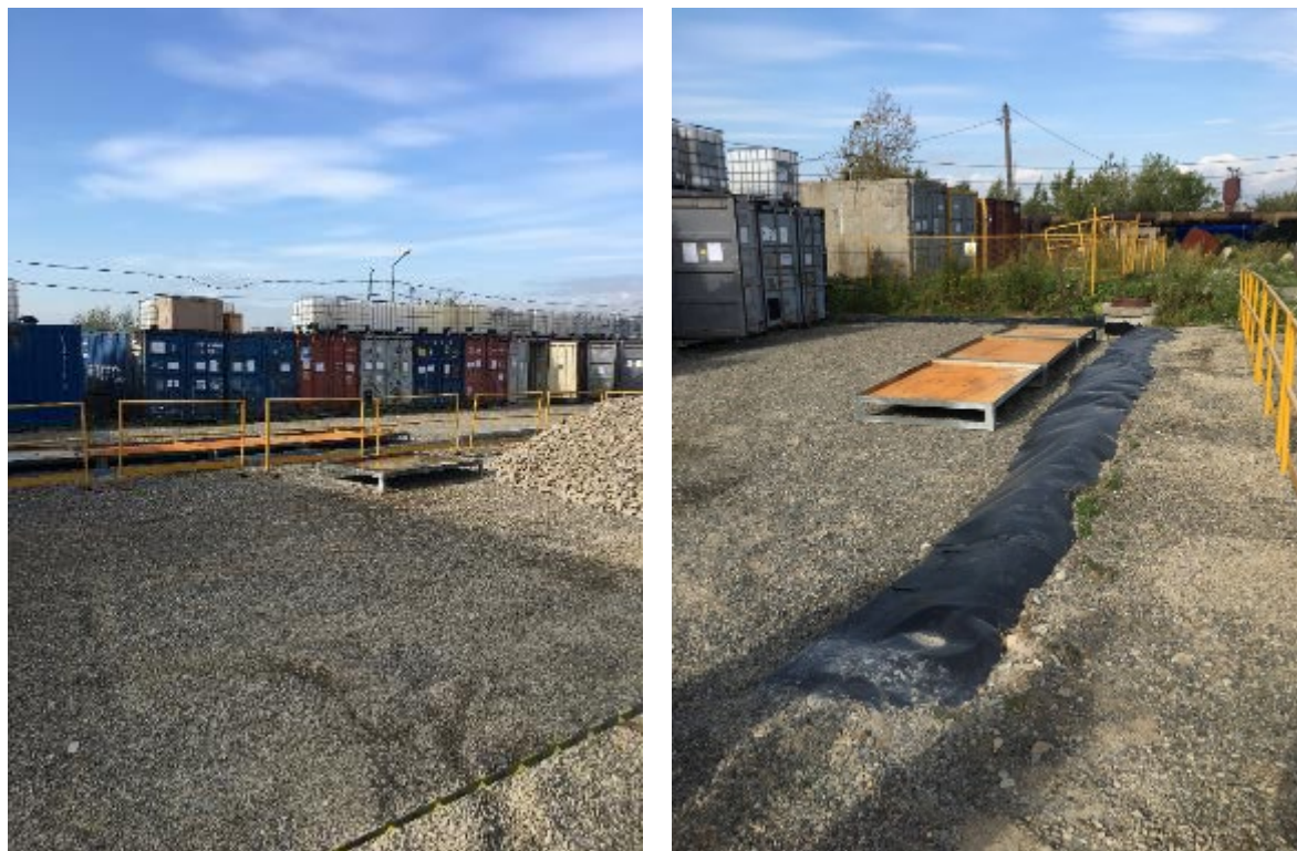
Figure 4.2 - Views across hazardous waste storage area (including trays for initial reception of drums and impermeable liner visible around the perimeter)
