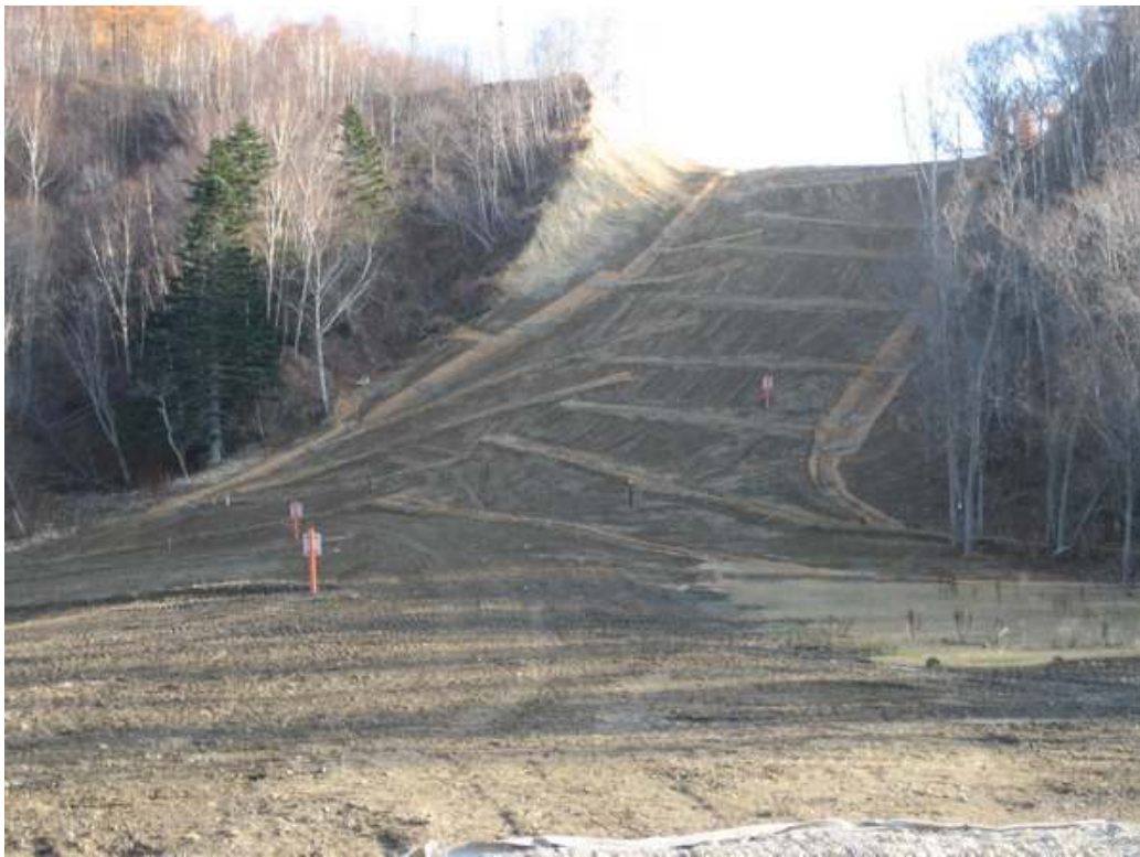
Photo 14 – KP 493 – Listvenitsa River Slope – Note the extensive armoured slope breakers on the slope.
