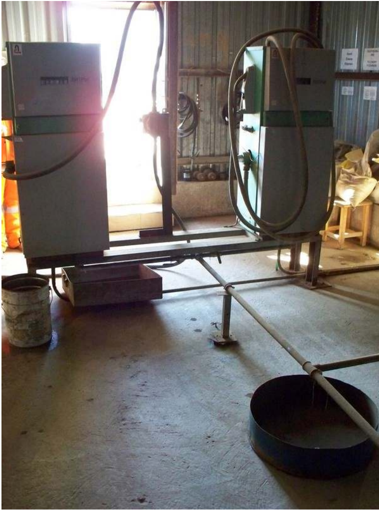
Photo 40 – Indoor diesel hand pumps at diesel storage area
