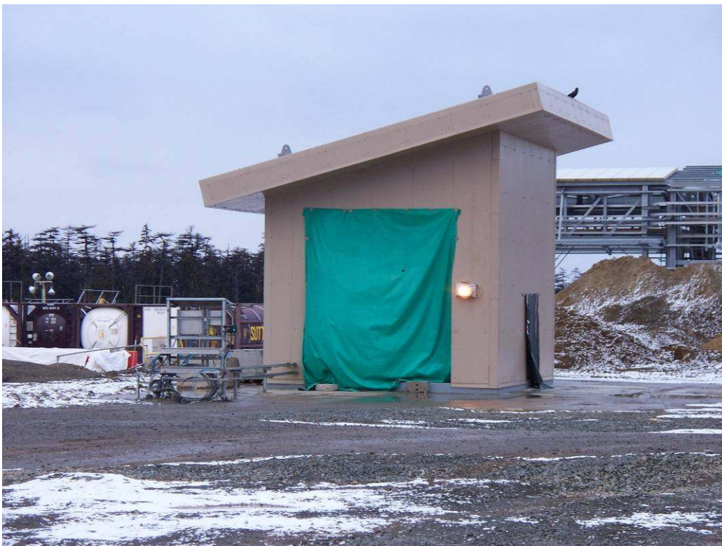
Photo 26 – Structure housing injection disposal wells – note tarpaulin-covered openings
