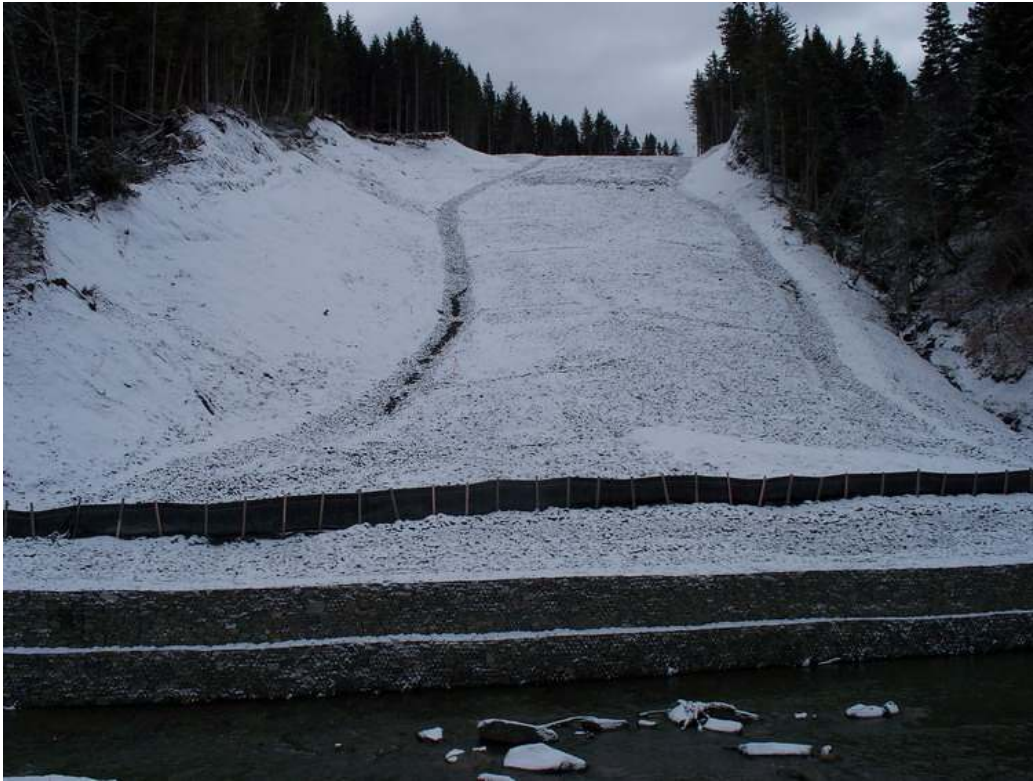
Photo 7 – Lesnaya 3 River Crossing and Slope – KP 376 – View south showing completed winterisation works on the slope including slope breakers and drainage. The riverbanks are protected with gabion walls.
