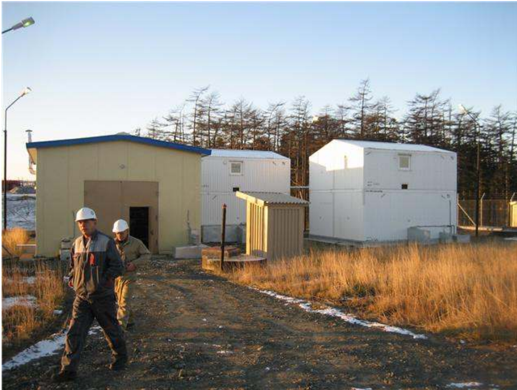
Photo 30 – Operations STP (for PAO and PMD)
