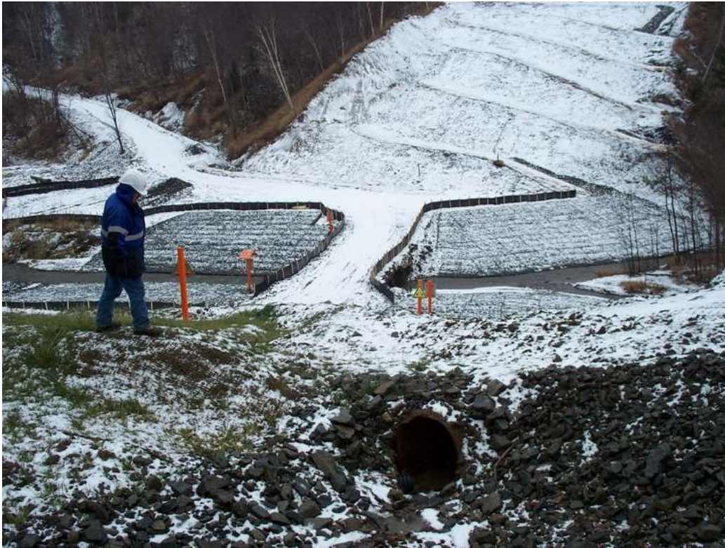
Photo 5 – Krinka River and Slopes – KP 348.5 – View south showing riverbank protection of reno mats and silt fences and both slopes with slope breakers. Note the growth of vegetation on the near slope, which was seeded early this year.
