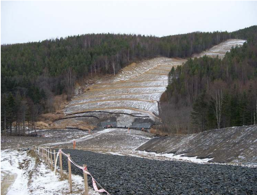
Photo 3 – Vidnaya River and Slope – KP 343 – View south showing armoured slope breakers and on going work on the riverbank. Photo taken from completed Fault Crossing No.11-14
