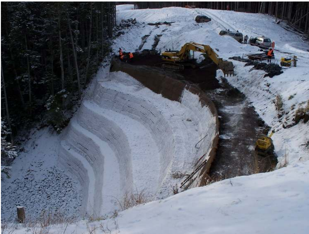
Photo 6 – Varvarka Ridge – KP 364 – Work in progress to stabilise the eastern slope of the ridge. The RoW is visible in the top of the photo.
