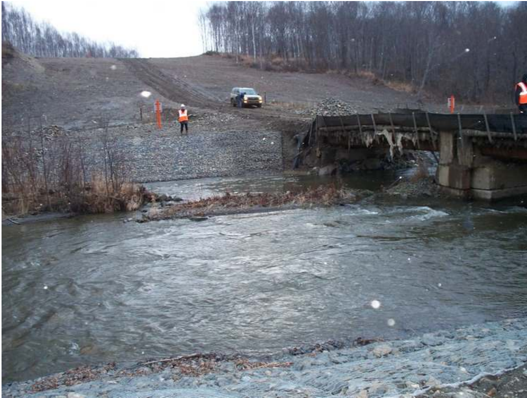
Photo 11 - Malakhitovka – KP 395 – The riverbanks are protected with Reno mats. The bridge and running track are still in place to provide access to the BVS.
