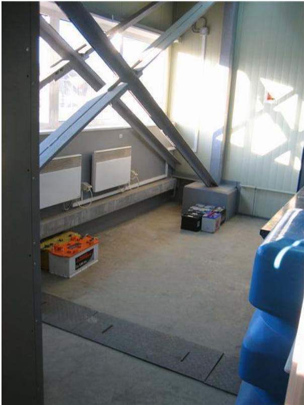
Photo 21 – PMD vehicle maintenance building: segregated battery storage area
