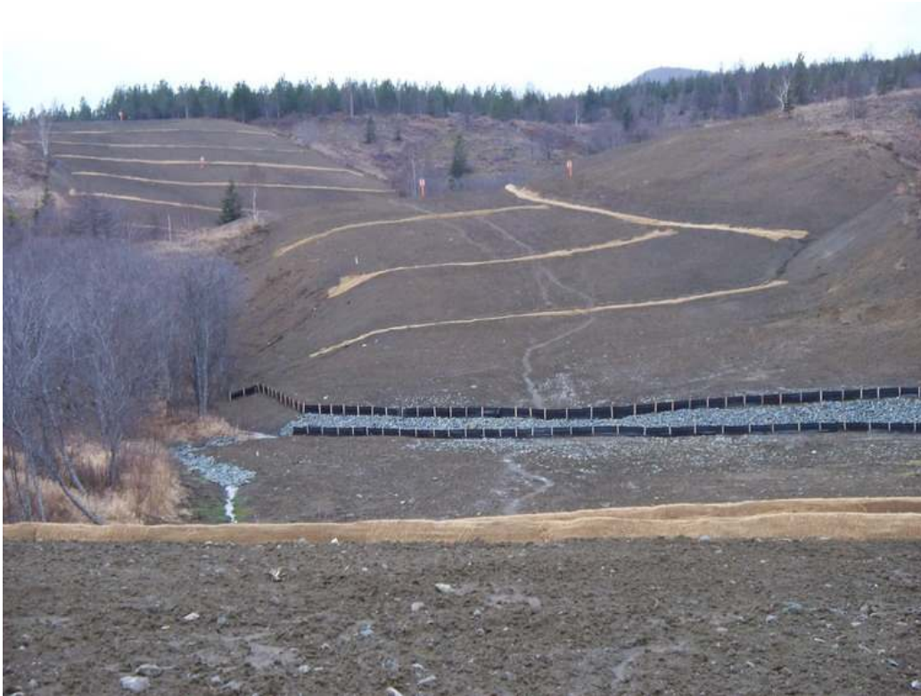
Photo 9 – Tura River – KP 409 – View across the river to the southern direction showing the riverbanks protected with riprap and partial coverage of erosion control on the opposite slope.
