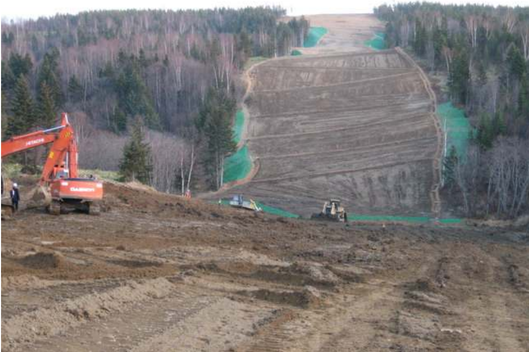
Photo 16 – KP 507.5 - On-going grading to contour at KP 507.5. Note the Rubulon Green geotextile on the side cuts of the opposite slope.
