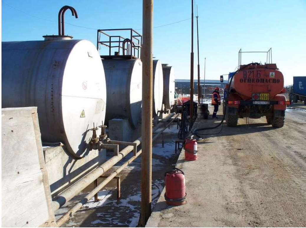
Photo 39 – Diesel storage area
