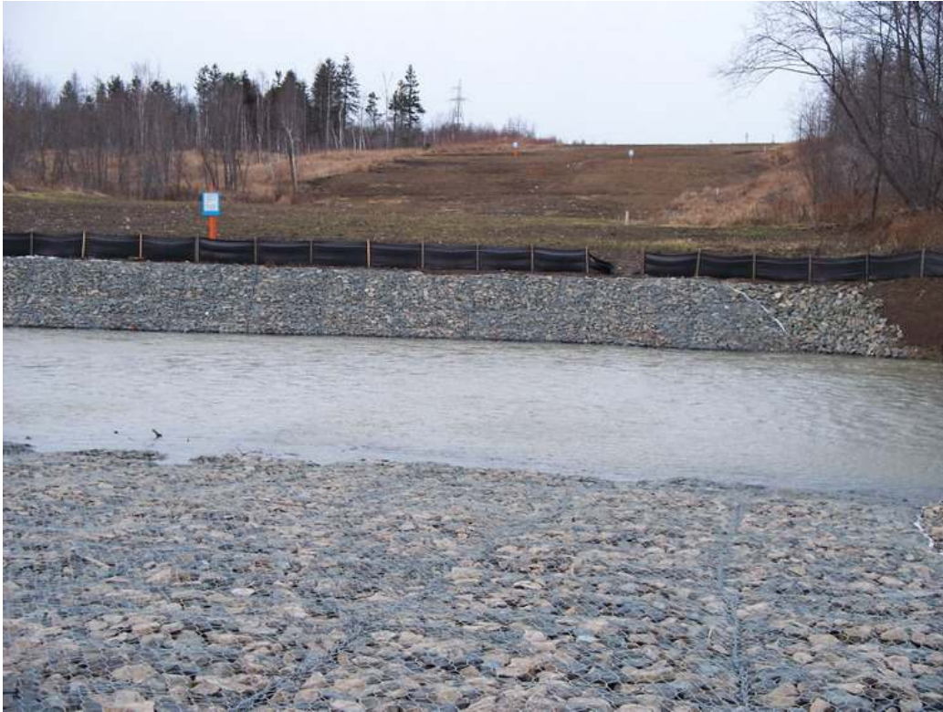
Photo 1 – Goryanka River – KP 313 – View to the north showing Reno mats on the banks and reinstated RoW beyond the sediment control above the bank.
