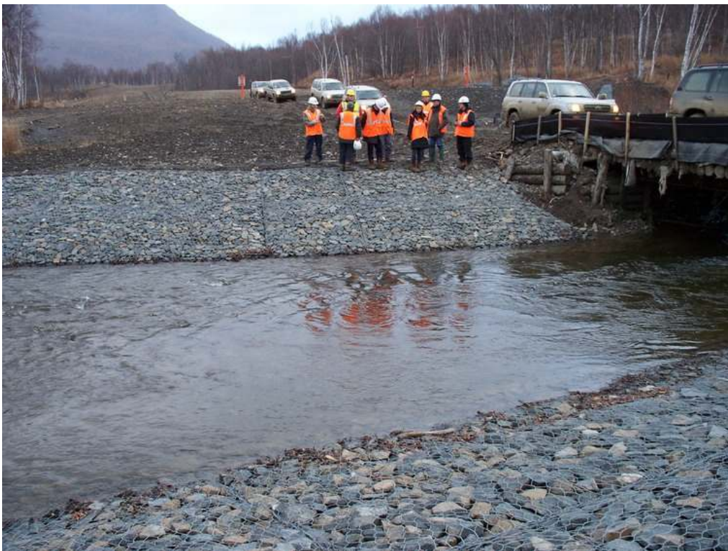
Photo 10 – Zvanka River – KP 391 – The riverbanks are protected with Reno mats. The bridge and running track are still in place to provide access to the BVS.
