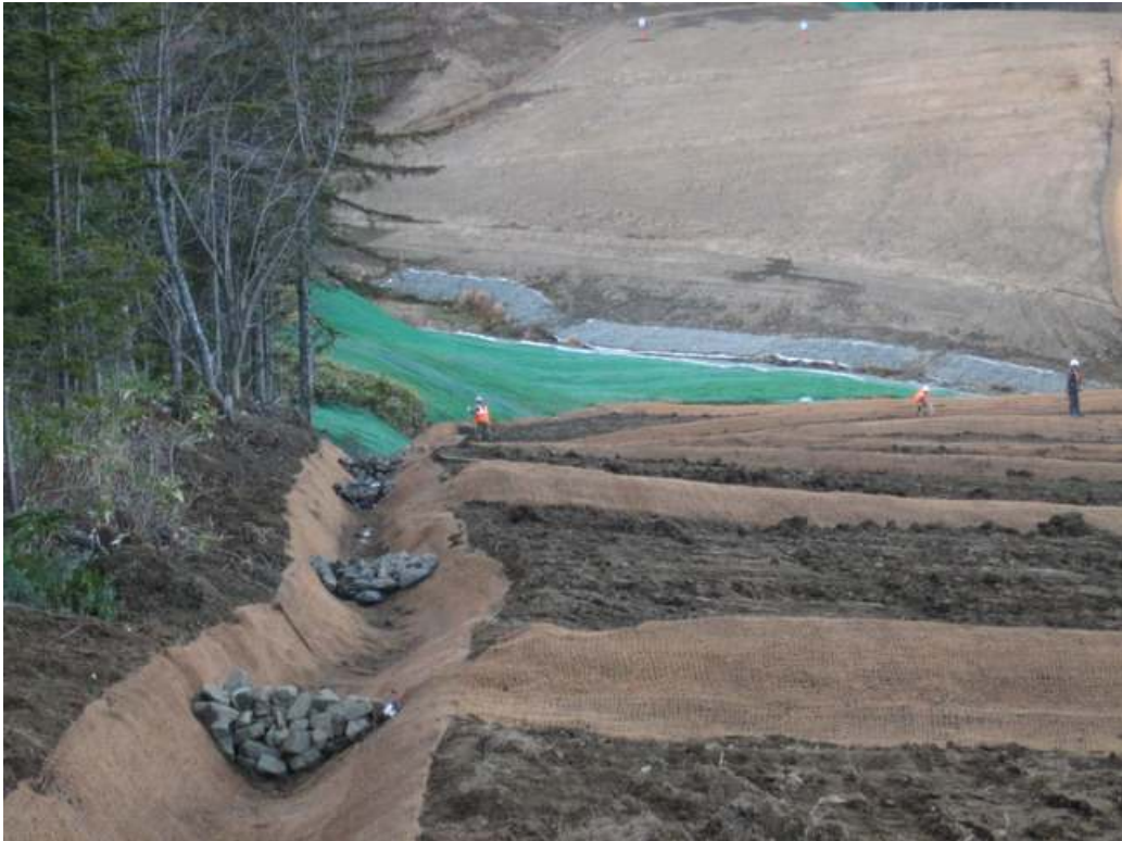
Photo 17 – KP 507 – Completed geojute armoured drainage and slope breakers on the near slope. Note the Rubulon Green geotextile on the lower side cut above the Reno matting.
