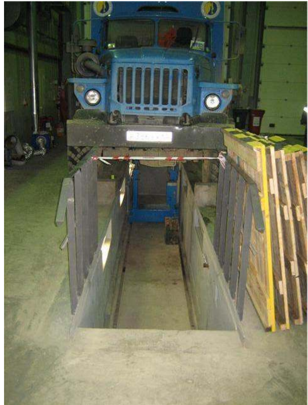
Photo 22 – PMD vehicle maintenance building: sub-floor work bay
