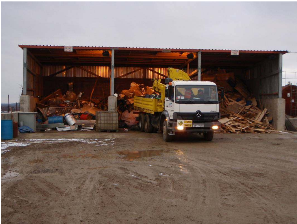
Photo 33 – Segregated waste storage bays at temporary waste transit area
