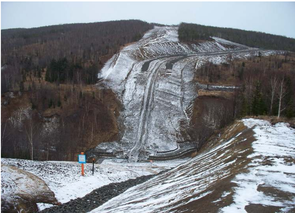
Photo 4 – Kormovaya River and Slopes – KP 347 – View to the north showing pending winterisation on the northern slope. Gabion wall on the riverbank is in the process of construction
