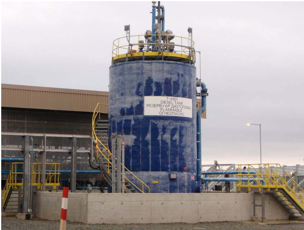
Photo 25 – Diesel storage tank within open bunded area – rain/melt water in drainage sump leads to multi-stage separator, through treatment system, into storm water overflow tank
