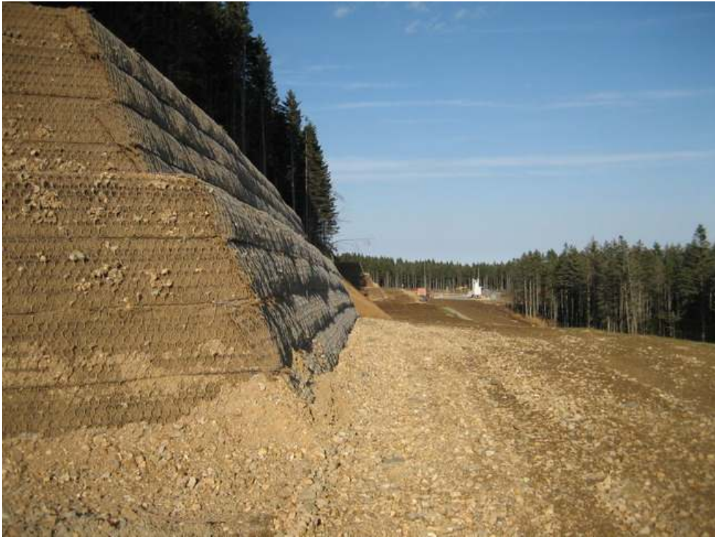
Photo 13 – RoW and stabilised sidewall at KP 483 – The sidewall is stabilised with Terra Mesh and gabion walls. The RoW is graded but with only temporary road to the BVS.
