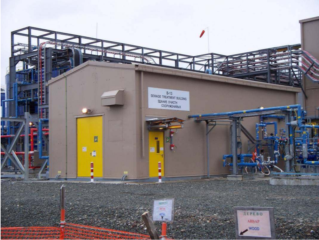
Photo 31 – OPF process facility STP, not used
