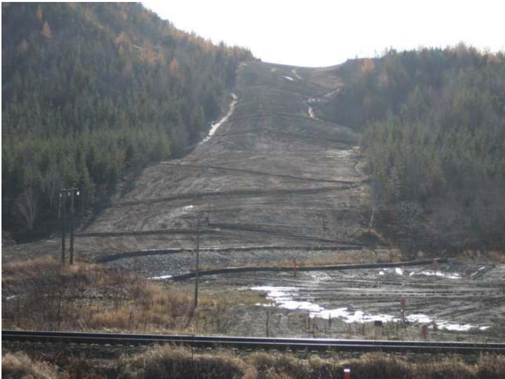
Photo 12 – KP 461 – Krasnaya River and Slope – view to the south showing the river protected with Reno mats and sediment control and the slope graded to contour and with drainage control.
