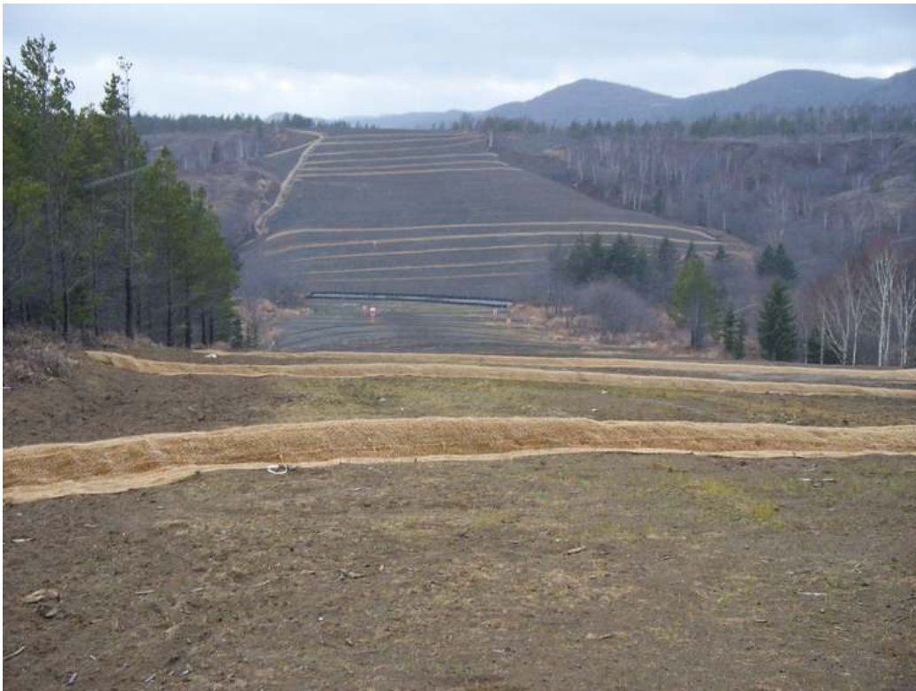
Photo 8 – Ssora River and Slopes – KP 407 – A view south showing the river with Reno matting and sediment control. The slopes on both sides of the river have armoured slope breakers and drainage.
