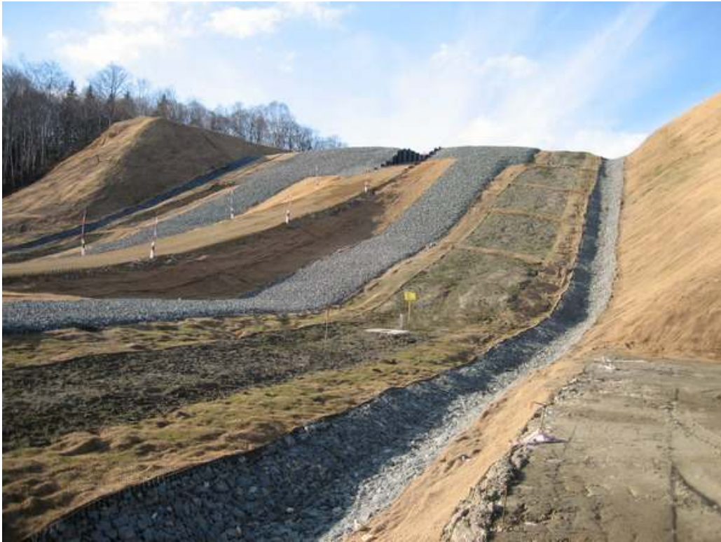
Photo 15 – KP 493 - Listvenitsa Fault – Completed fault crossing works. Note the feathered back side cuts with geojute protection.
