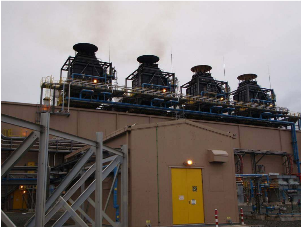
Photo 32 – Power generation turbines: A-4001C/D (left of picture) currently on diesel, and gas turbines A-4001A/B (right of picture) due to be commissioned November 2008
