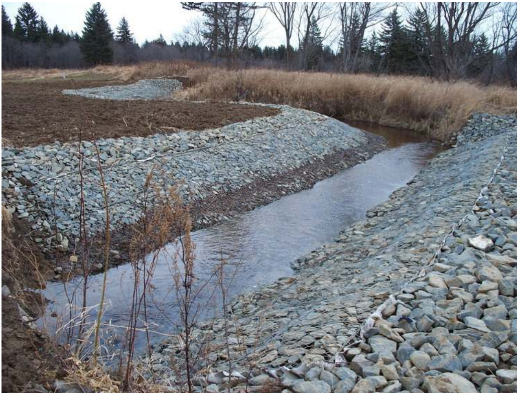
Photo 2 – Klinovka River – KP 317 – View of the riverbanks protected with Reno matting at the crossing and at the meander adjacent to the RoW. Also, note the graded RoW beyond the banks.
