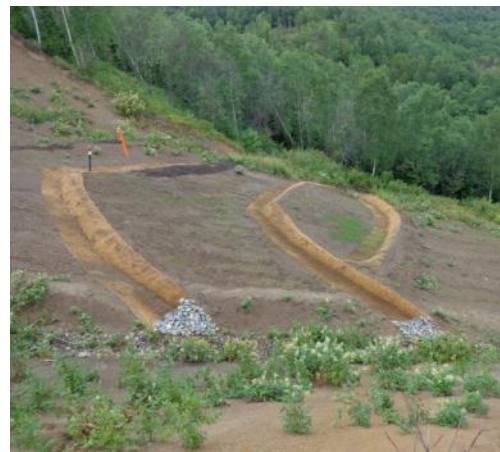
Photo 9 R. Kormovaya showing slope failure (2011) and repair works (2012)
