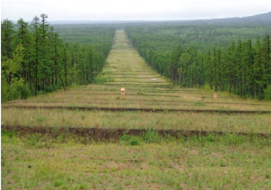
Photo 7 Sandy slope at KP128 showing improved vegetation cover
