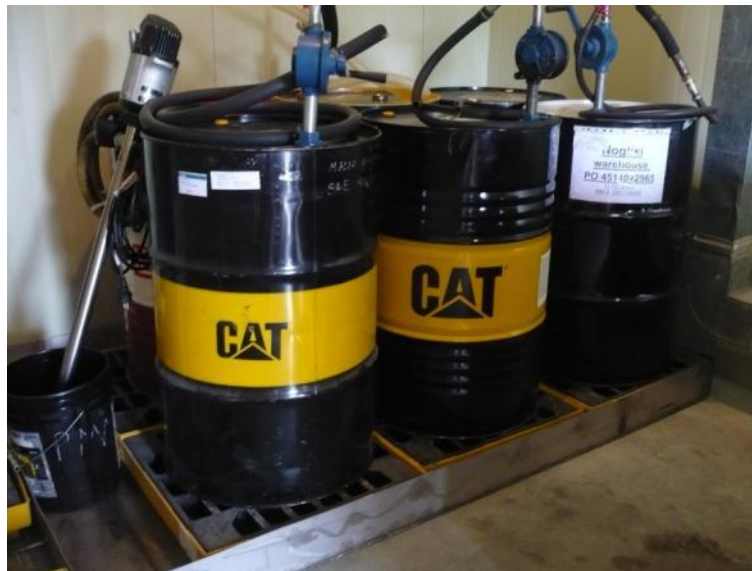
Photo 17 Secondary containment of oil drums at Nogliki PMD
