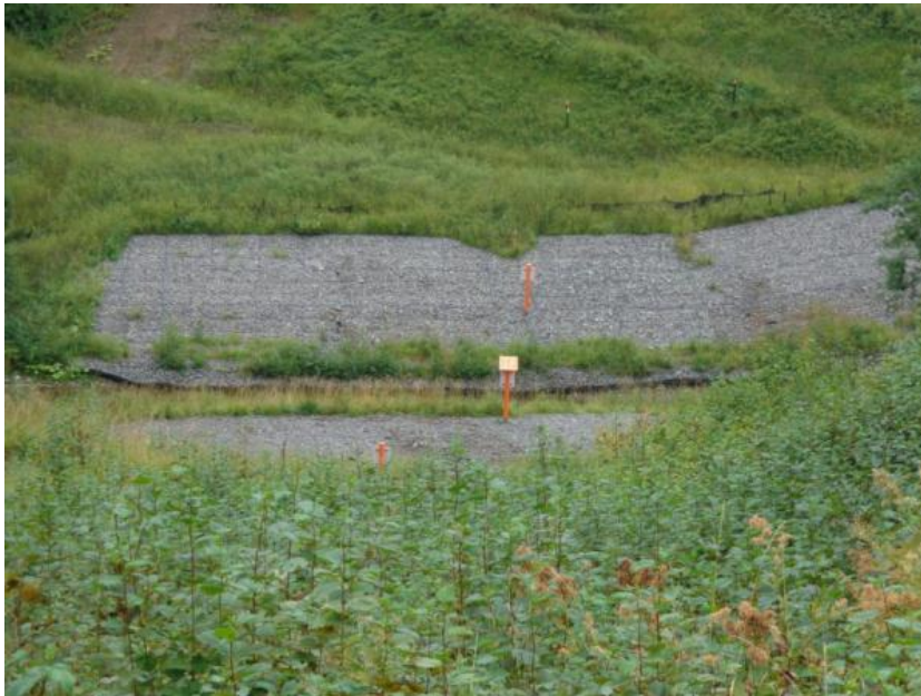
Photo 11 Slopes of the R. Krinka showing dense vegetation on geojute fortified slope breakers
