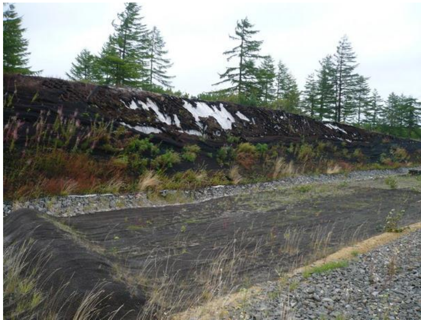
Photo 13 Failure of geonetting at Fault Crossing 1
