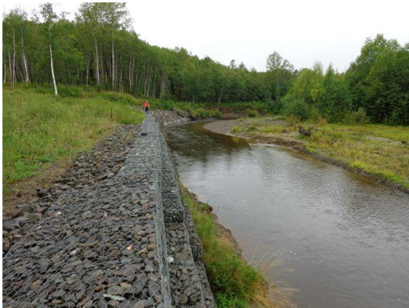
Photo 16 Gabion wall on the south bank of the R. Pobiedinka
