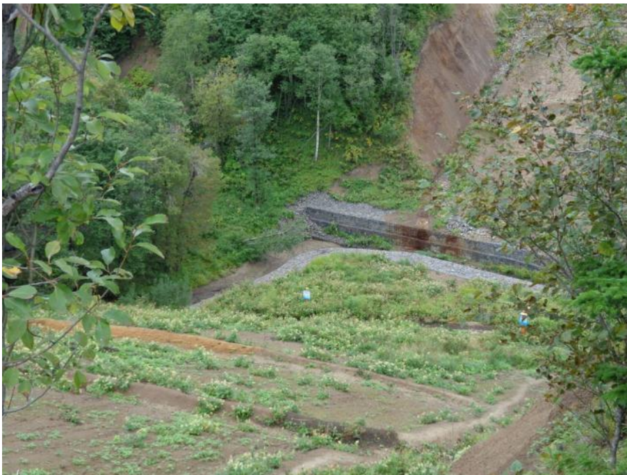
Photo 15 Slopes adjacent to R. Kormovaya with repairs to silt fencing required
