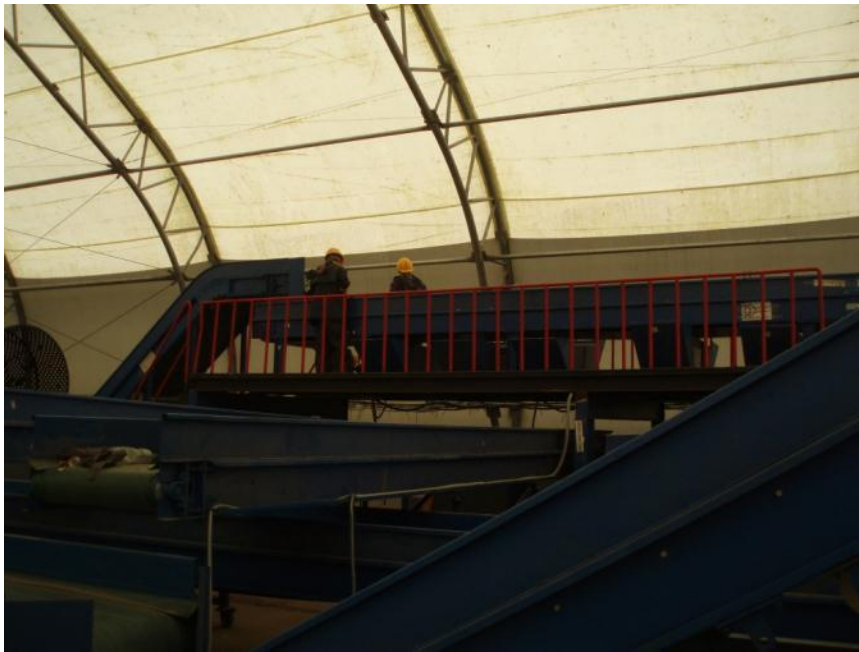
Photo 23 Waste segregation facilities at the Korsakov landfill
