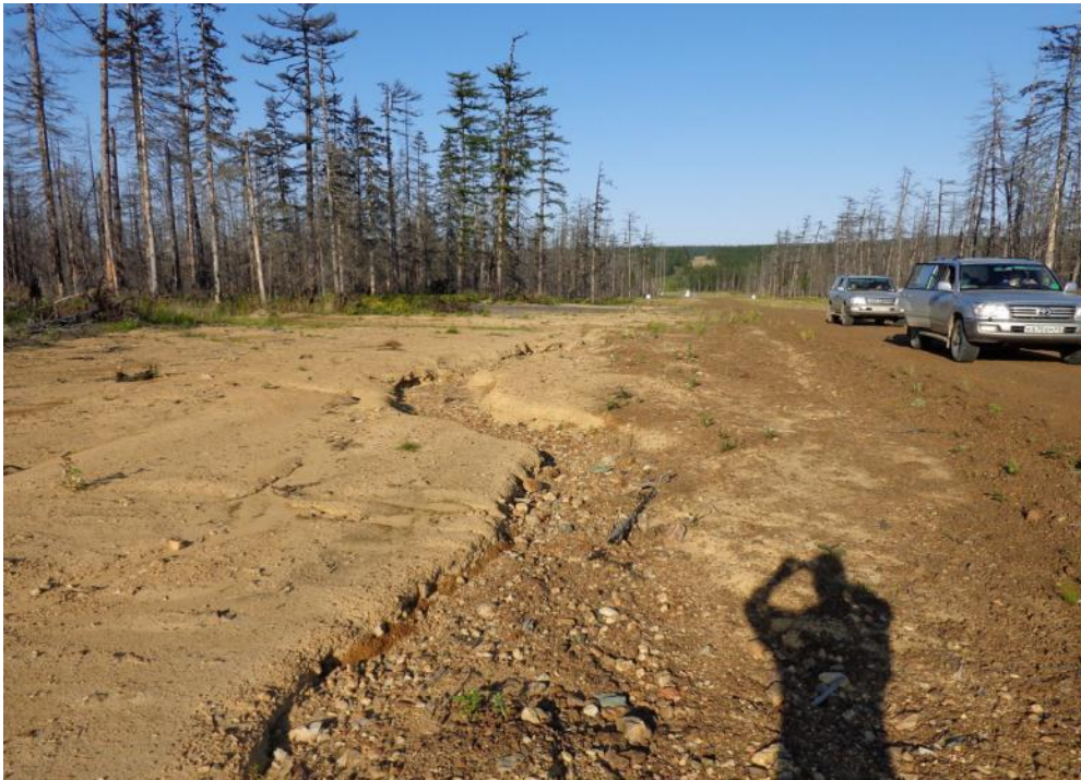
Photo 10 RoW at KP15 showing development of erosion
