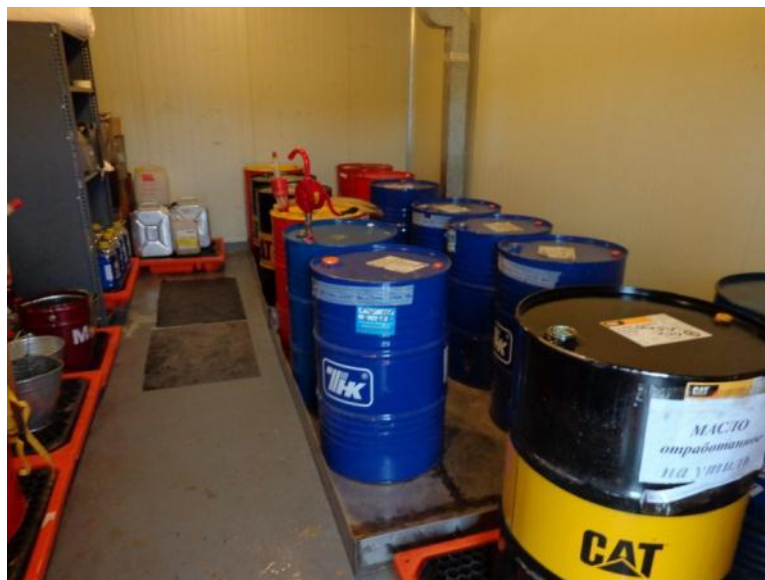
Photo 19 View of drums in large secondary containment tray
