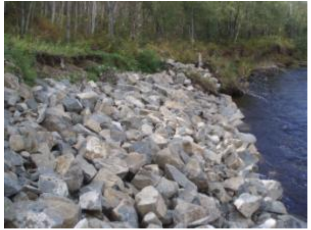
Photo 4 – New rip-rap installation
