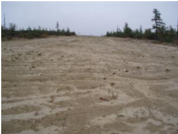
Photo 3 – Slopes breakers on the approach to the river
