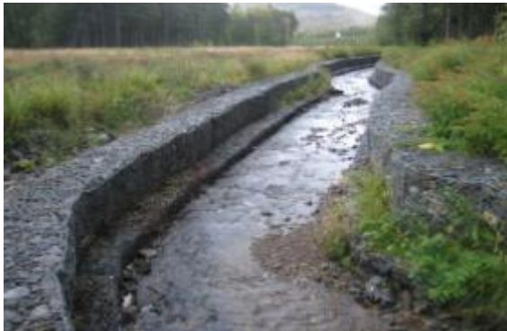
Photo 3 – View of the river crossing with riprap lined channel and good re-vegetation.
