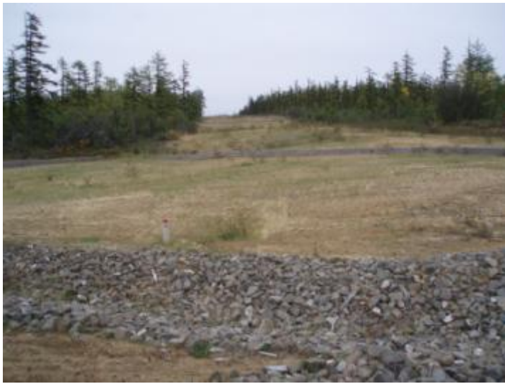
Photo 1 – Armoured drainage ditch in good condition
