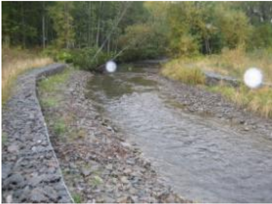
Photo 1 – View upstream of the river crossing showing Reno matting and gabion walls.
