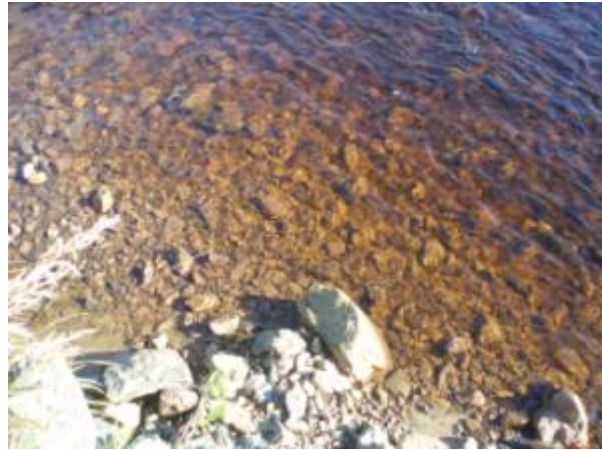
Photo 2 – Scour upstream on east bank
