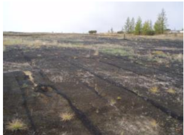
Photo 4 – Washout behind Slope Breaker
