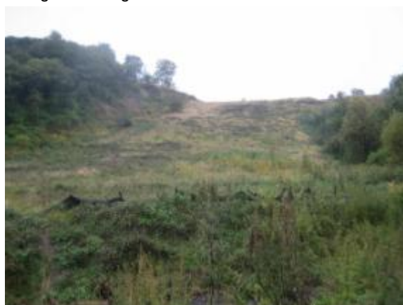
Photo 6 – View of a RoW slope north of the Nitui with good re-vegetation
