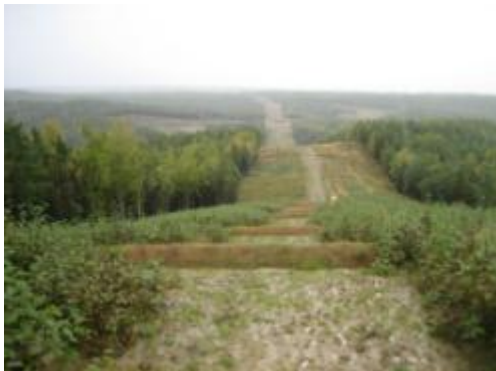
Photo 3 – A close up view of the fortified slope breakers and tree saplings on the slope.
