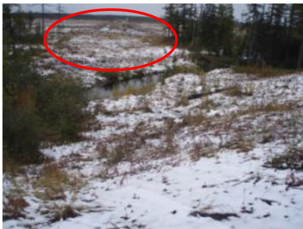
Photo 1 – Bank protection and vegetation (note visible pipeline crowns)
