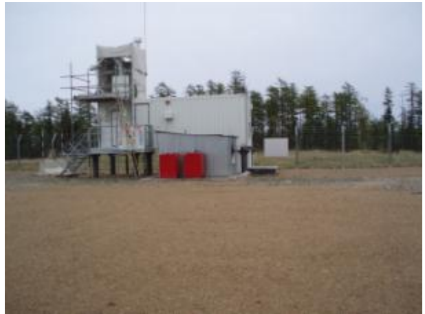
Photo 2 – Temporary diesel generator and fuel day tank (note rudimentary containment)
