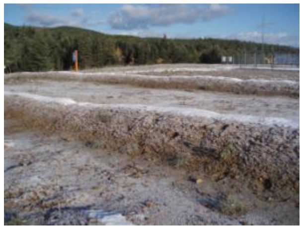
Photo 4 – Slope breakers with evidence of siltation
