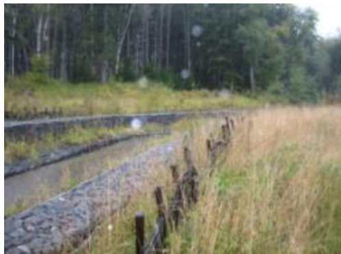
Photo 1 – View upstream showing Reno matting and gabion walls. Also note the dense vegetation.
