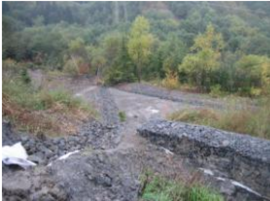
Photo 1 – View gabion walls and drainage channels.
