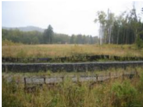
Photo 3 – View of RoW to the south of the crossing showing dense re-vegetation.
