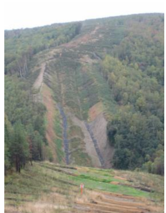
Photo 2 – View to the south showing a partially vegetated south slope. The slope is covered in green vegetation and brown soil, with a road visible in the foreground.
