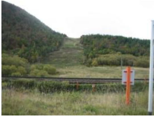
Photo 1 – View to the south showing well vegetated slope and river crossing
