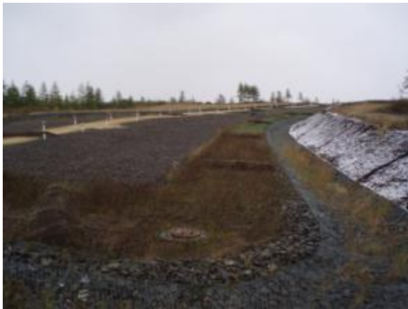
Photo 3 – Failing side cut
