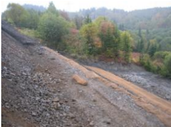
Photo 3 – View of terracing and geotextile during on going work.
