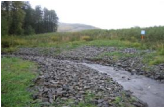
Photo 3 – View of the river crossing with riprap lined channel and good re-vegetation.
