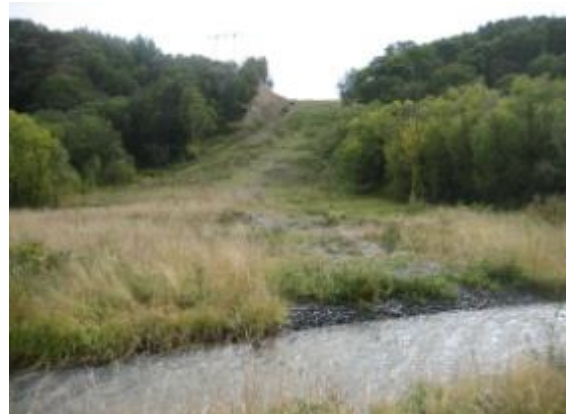
Photo 2 – View south showing vegetated south slope with an erosion channel on the east side .
