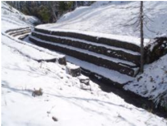
Photo 1 – Gabion engineering at toe of slopes
