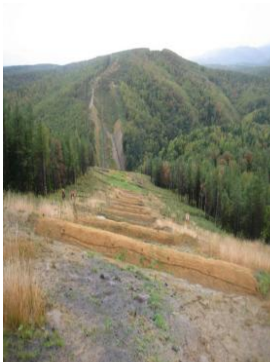
Photo 1 – View to the south of vegetated RoW with fortified slope breakers on the access track.
