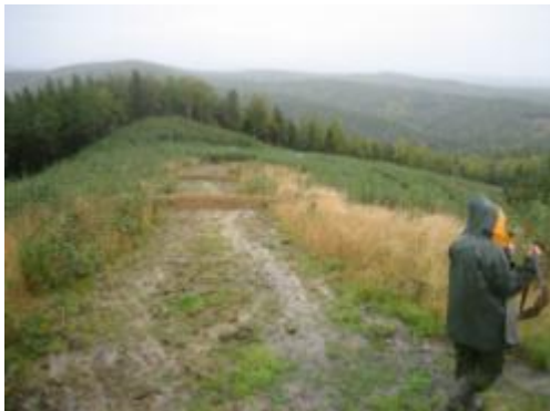
Photo 3 – A close up view of the fortified slope breakers and tree saplings on the slope.
