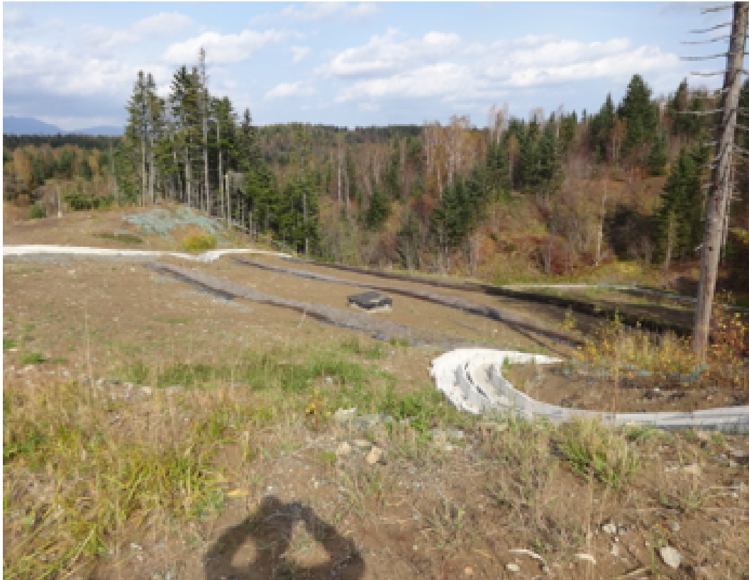
Photo 11 - View to the east from the RoW at KP 514 showing a Category 3 geotechnical repair work on a landslide
