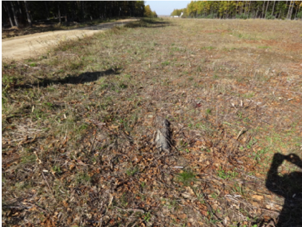
Photo 1 – KP 64 – RoW section with high concentration of tree saplings cut by manual means. Note the grass in place
