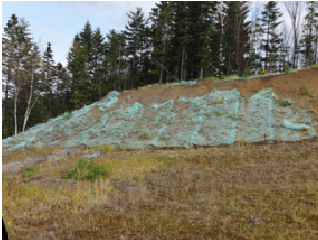
Photo 10 - View of one of the side cuts in the vicinity of KP 514 showing deteriorating geojute and bare side cut
