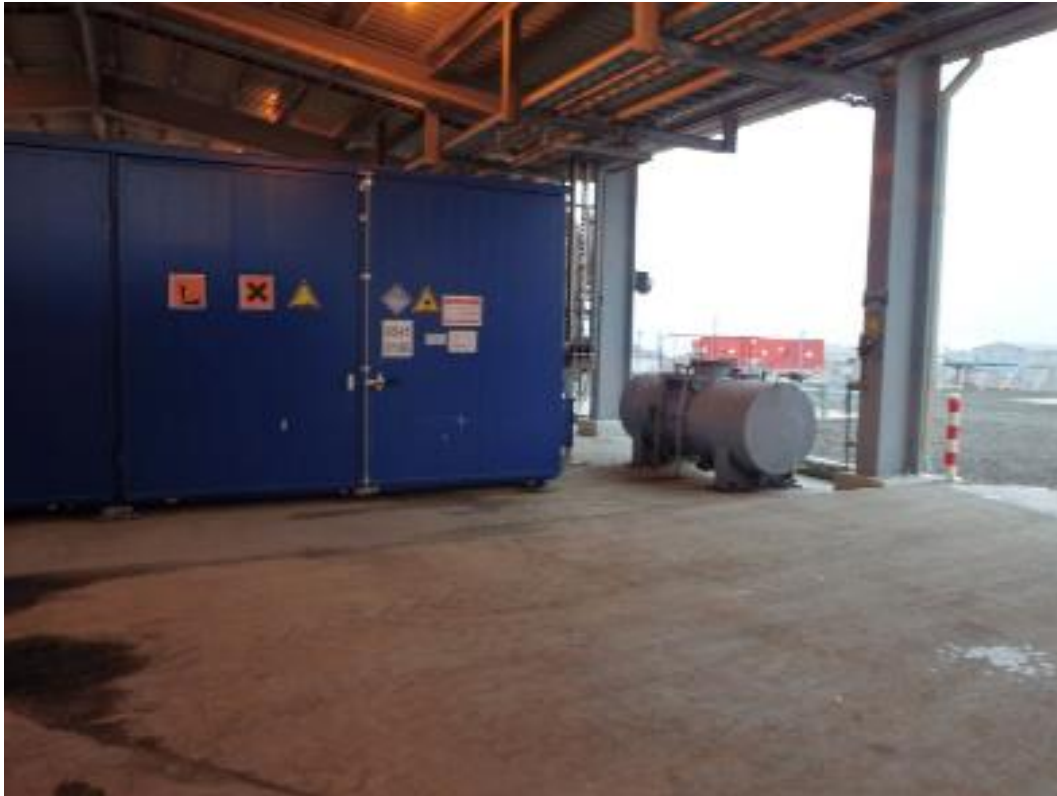
Photo 12 - Main chemical storage area at OPF
