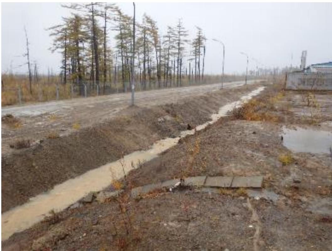
Photo 23 - Silt-laden storm water discharging off-site without treatment
