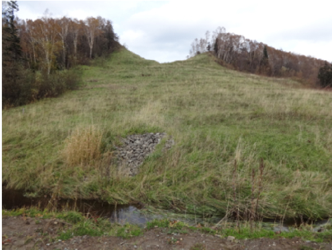
Photo 4 - KP 510.5 - Sovietskoy Ridge - Steep slope with good slope breakers and vegetation cover
