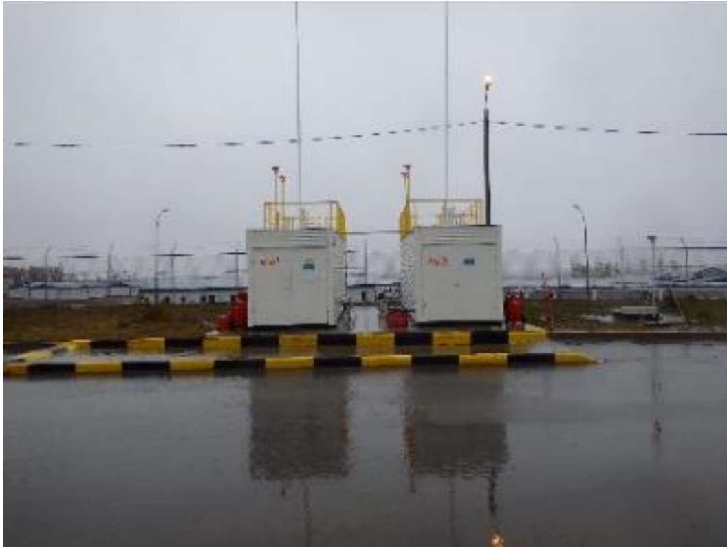
Photo 15 - Refuelling area at OPF PMD
