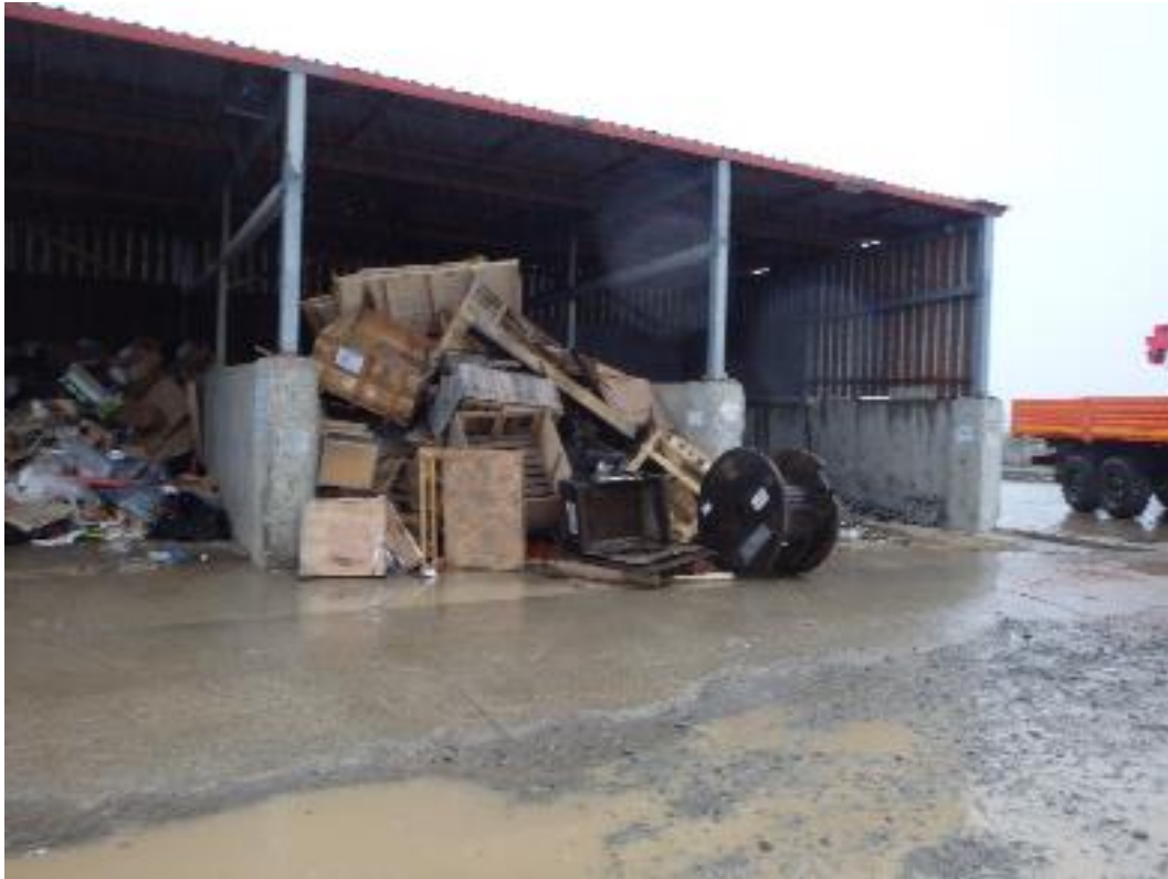
Photo 18 - Non-hazardous waste storage bays at OPF Waste Transit Area
