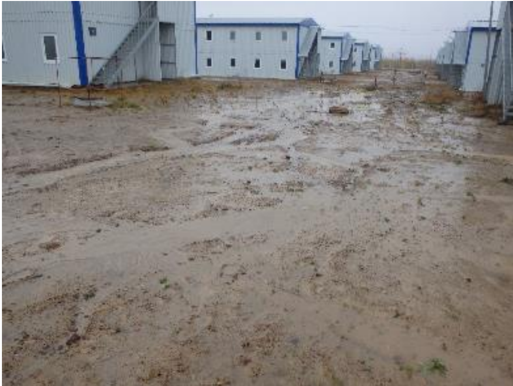
Photo 22 - Fly camp area under renovation - poor drainage and erosion control
