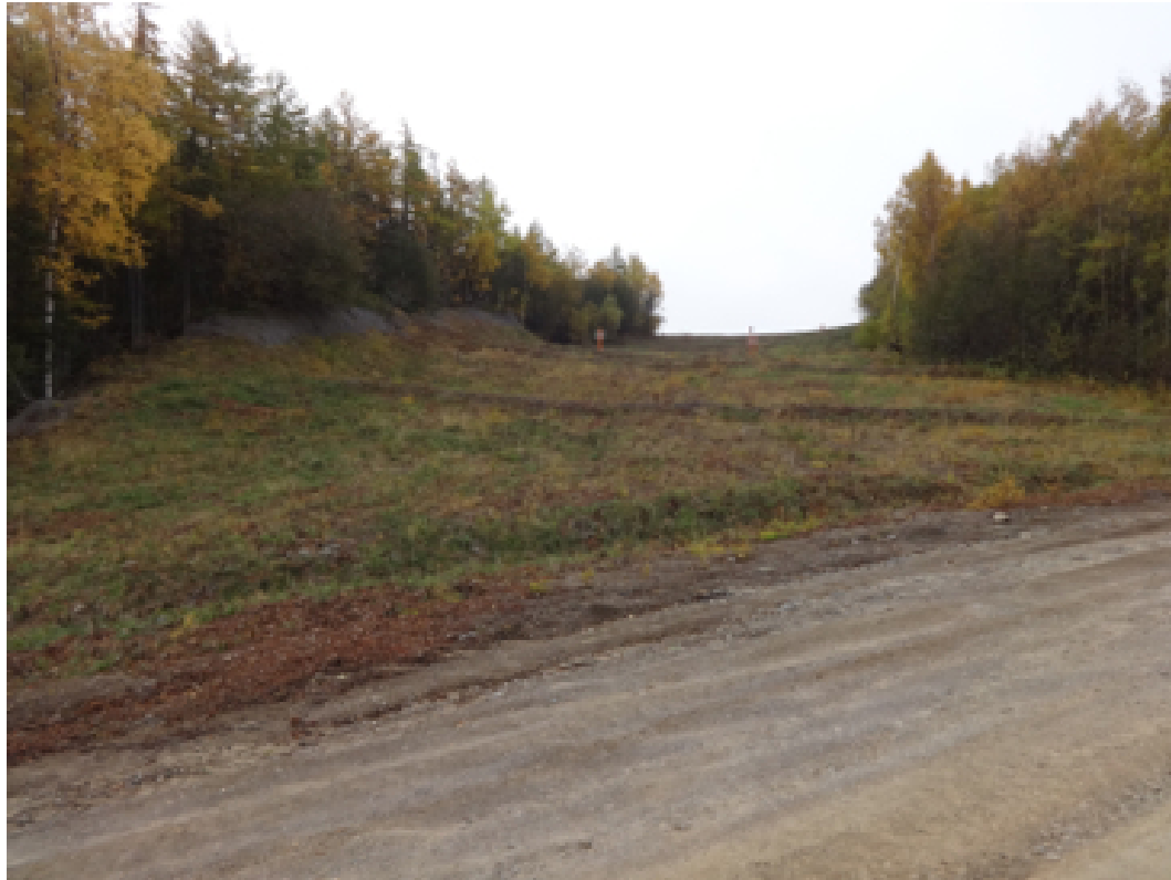
Photo 8 - KP 97 showing steep slope with slope breakers
