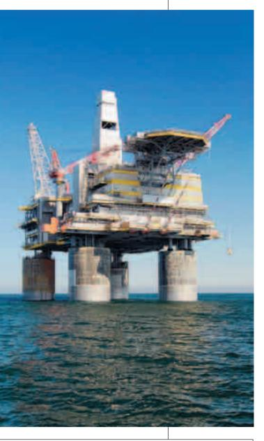
The LUN-A gas production rate is up to 10 million cubic metres of gas per day per well. It means that the gas amount supplied by each of the LUN-A wells can feed a 2GW power plant at full operation.
